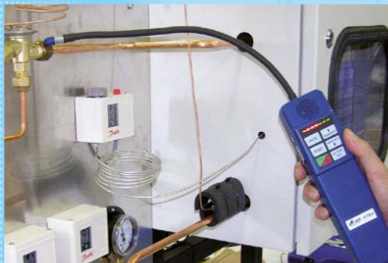
Leak testing at expansion valve
