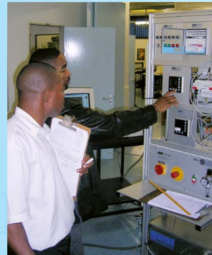
Setting on a digital controller
