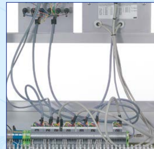
Industry-standard, flexible cabling
